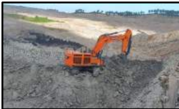
Gambar 4.1 Excavator Doosan PC-800 HE
