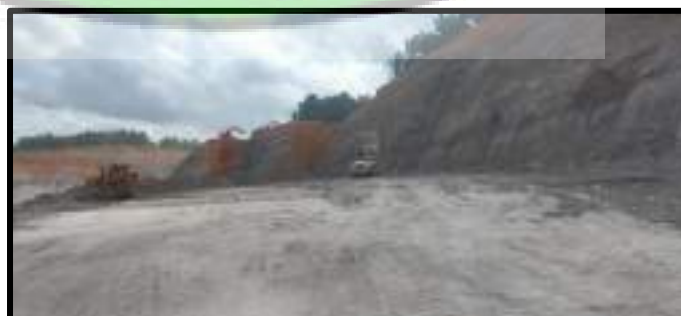
Gambar 4.8 Kondisi Dumping Point
